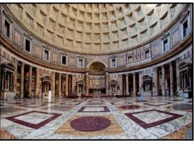
Detail of the **Roman Pantheon** interior. The dome ceiling consists of coffered concrete patterns.
